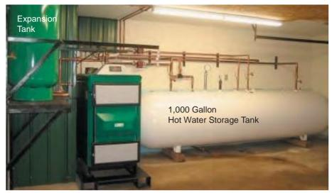
EKO 60 with 1,000 gallons of pressurized hot water storage and expansion tank.
